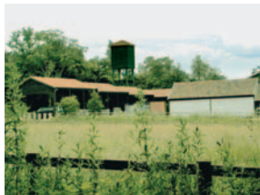
Left: Base station equipment for all mobile network operators is concealed in a specially designed watch tower in Epping Forest.
